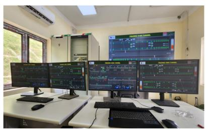
The open standard SCADA system communicates using industry standard protocols such as Modbus TCP and Siemens IP-ISO S7 protocol ensuring future interoperability with any automation equipment manufacturer. Today the system already monitors above 20 000 parameters and could allocate up to 65 000 tags in the future thanks to its open architecture concept.
